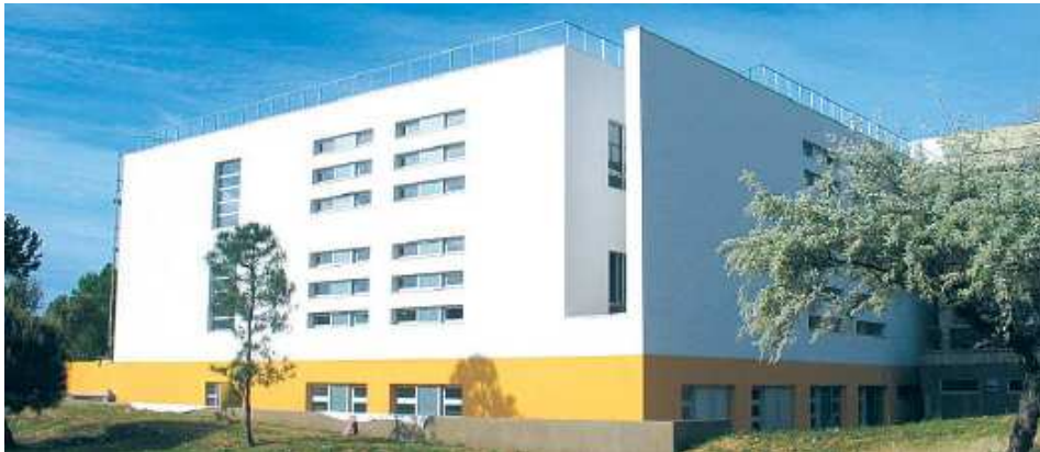
West and North façades
